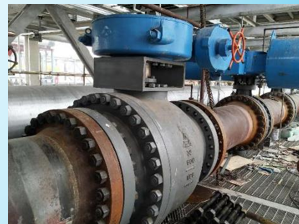
Ningxia Baofeng Energy Synthetic Device Synthetic Boundary Main Manual Valve May.2020
