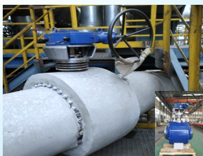
China Shenhua Coal-to-Liquid Chemical Co., Ltd. Ordos Coal-to-Liquid Bureau High Temperature Oil-coal Slurry Shut-off Valve Replace German HARTMANN Ball Valve March.2015
