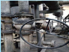
Shandong Jinmei Riyue Chemical Co., Ltd. Black and Grey Water Shut-off Valve Sept.2018
