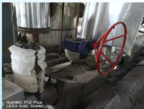
Inner Mongolia Yitai Coal Co., Ltd. Chilling Water Pump Shut-off Valve Sept.2018
